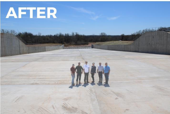
Clear Creek Spillway construction began in November 2020, and the Phase One 9.9-million-dollar investment is recently completed, with a Phase Two dam evaluation study to be complete by end of May 2022. The new spillway holds over 100 tons of steel and is more than two football fields in length.
