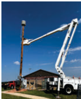
New storm siren installation at Abe Raizen Park
